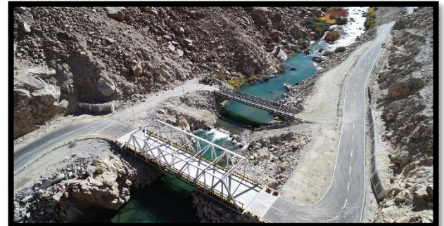
Bridge on DSDBO Road Ladakh
